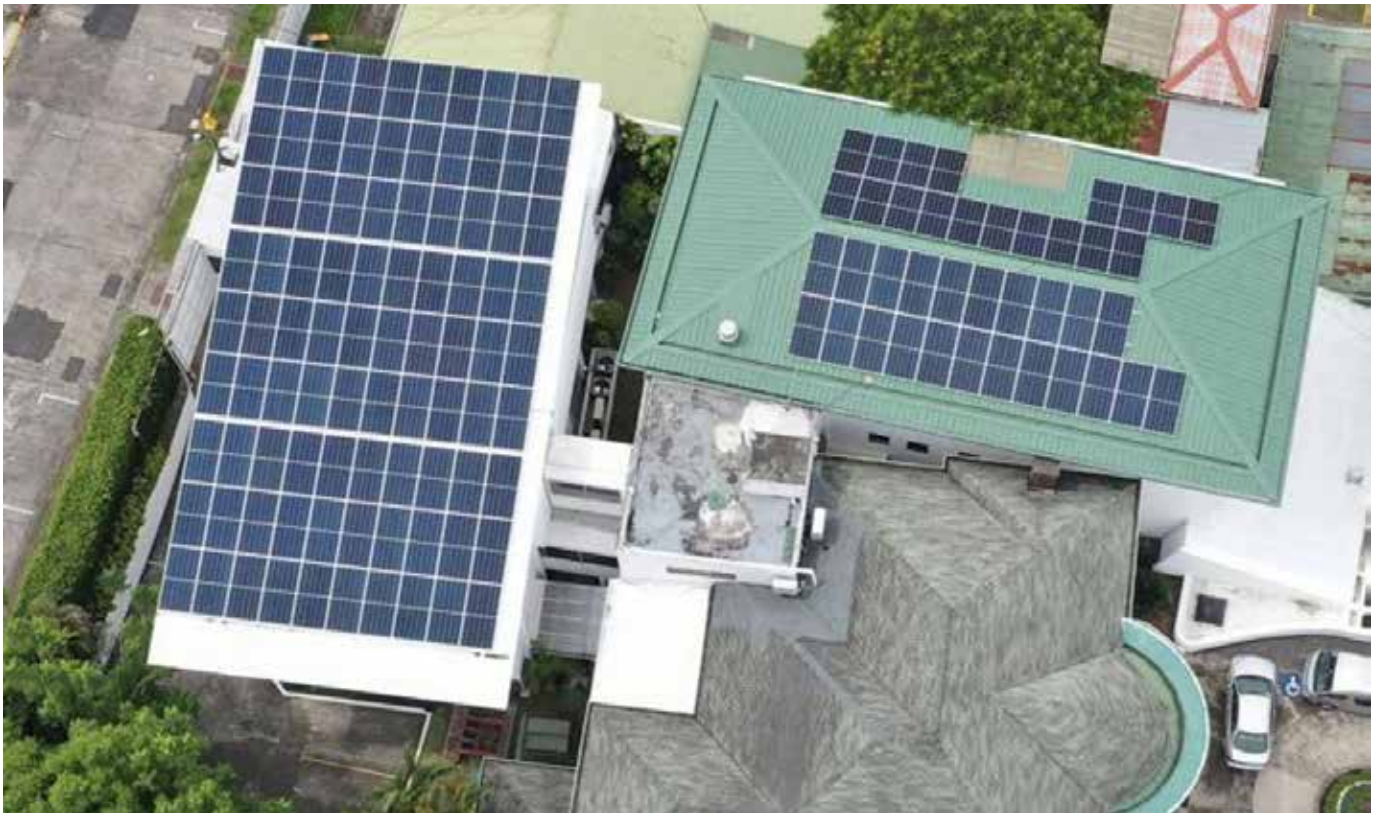
Aerial view of the solar panels installed on the premises of the Court.
